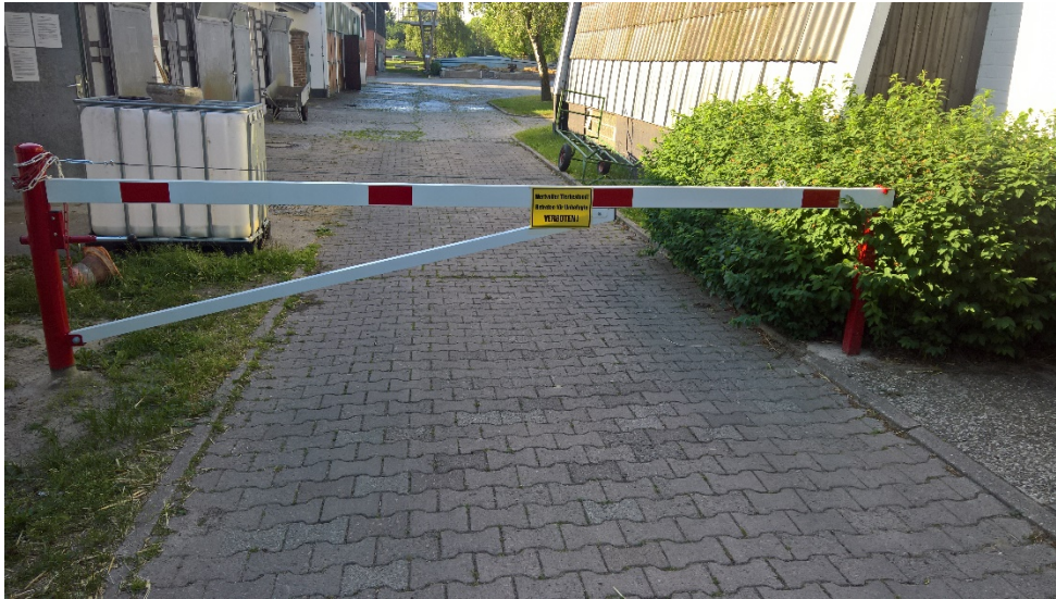
Figure 14: Example of a barrier for restricting and steering vehicle traffic.
